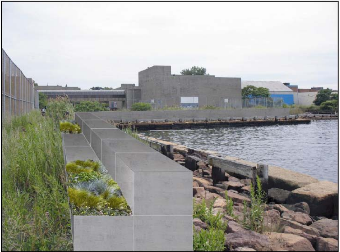
Figure 2: Conceptual modular sea wall design protection for a school and community center in East Boston.
